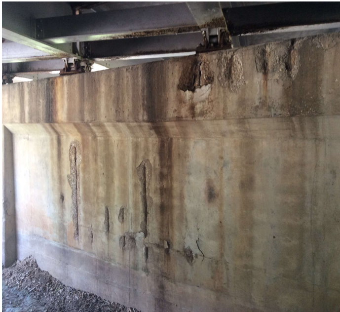
PHOTO 1 Description NB lanes bent 5 ahead side spalling to pier wall and cap with steel exposed.
