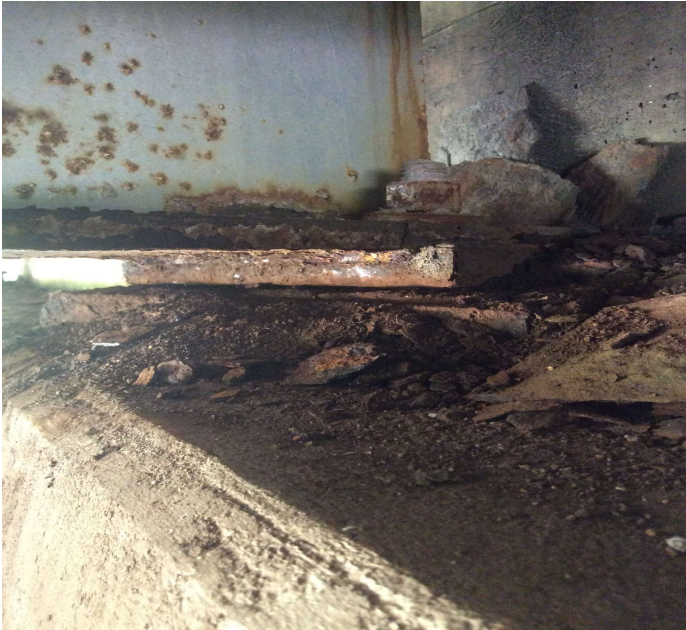
PHOTO 3 Description Abutment 2 bearing 2 is free floating and is moving when under load.
