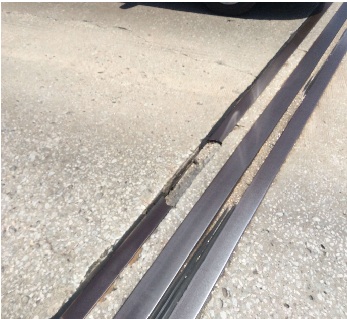
PHOTO 1 Description SB lanes abutment 2 road iron Missing.
