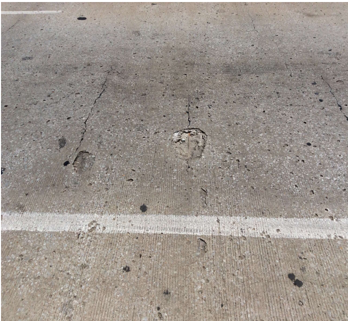
PHOTO 3 Description Span 2 SB lanes left lane spalling with steel exposed approximately 7' from bent 1 road iron.
