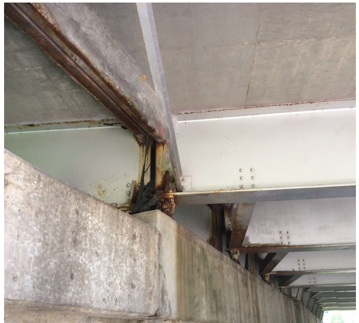
PHOTO 2 Description NB lanes span 5 bent 4 end of beam corrosion.
