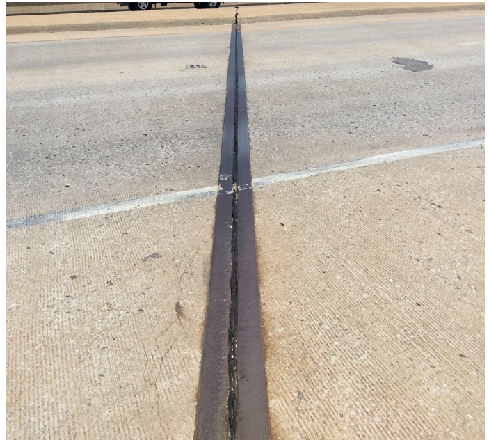
PHOTO 2 Description SB lanes bent 5 joint material
