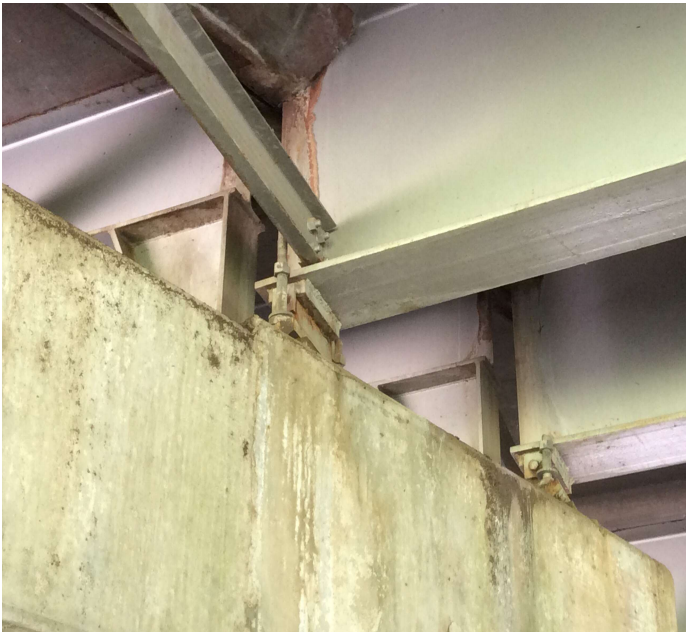
PHOTO 1 Description Typical anchor bolts with excessive projection.
