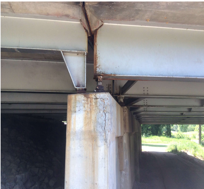
PHOTO 1 Description NB lanes Bent 1 right column 6 cracking with delaminated areas.
