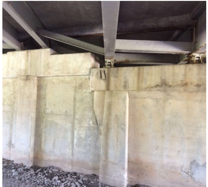
PHOTO 2 Description NB lanes bent 5 behind side spalling with steel exposed above column 4.
