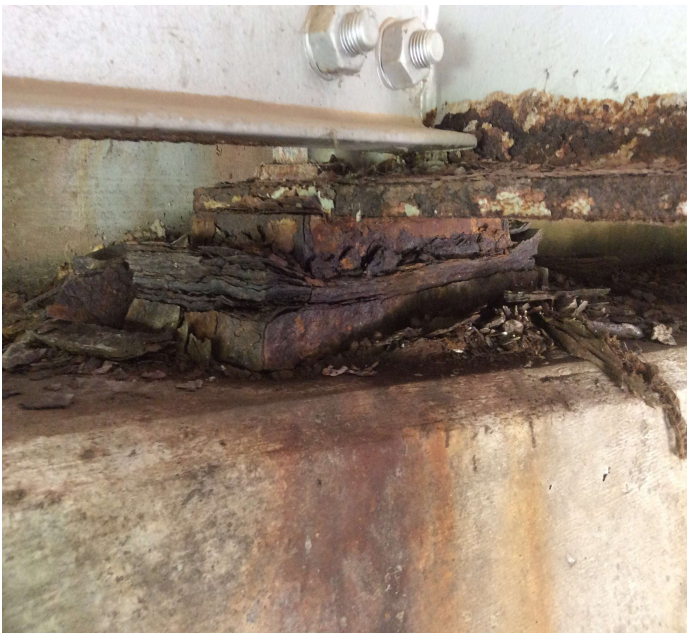
PHOTO 1 Description Typical view of bearings at Abutment 2 SB lanes
