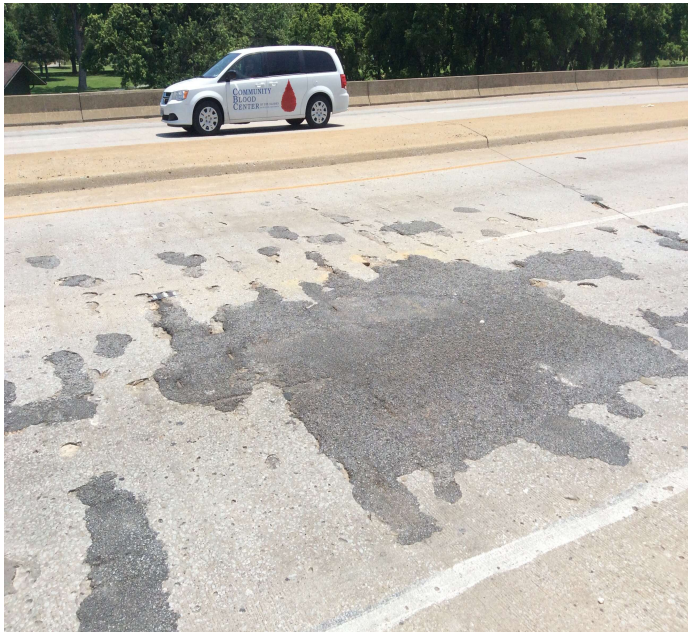
PHOTO 1 Description Area with spalling, patching and steel exposed in SB lanes adjacent bent 2 in span 3
